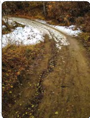
EROSION CAUSES AN UNEVEN TRAIL SURFACE
