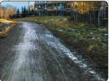
NEGATIVE CROSS DRAINAGE RESULTING IN SLIPPERY CONDITIONS AND EROSION AND POTENTIAL FOR WINTER ICING
