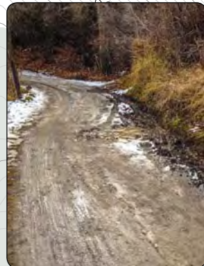
NEGATIVE CROSS DRAINAGE RESULTING IN SLIPPERY CONDITIONS AND EROSION AND POTENTIAL FOR WINTER ICING
